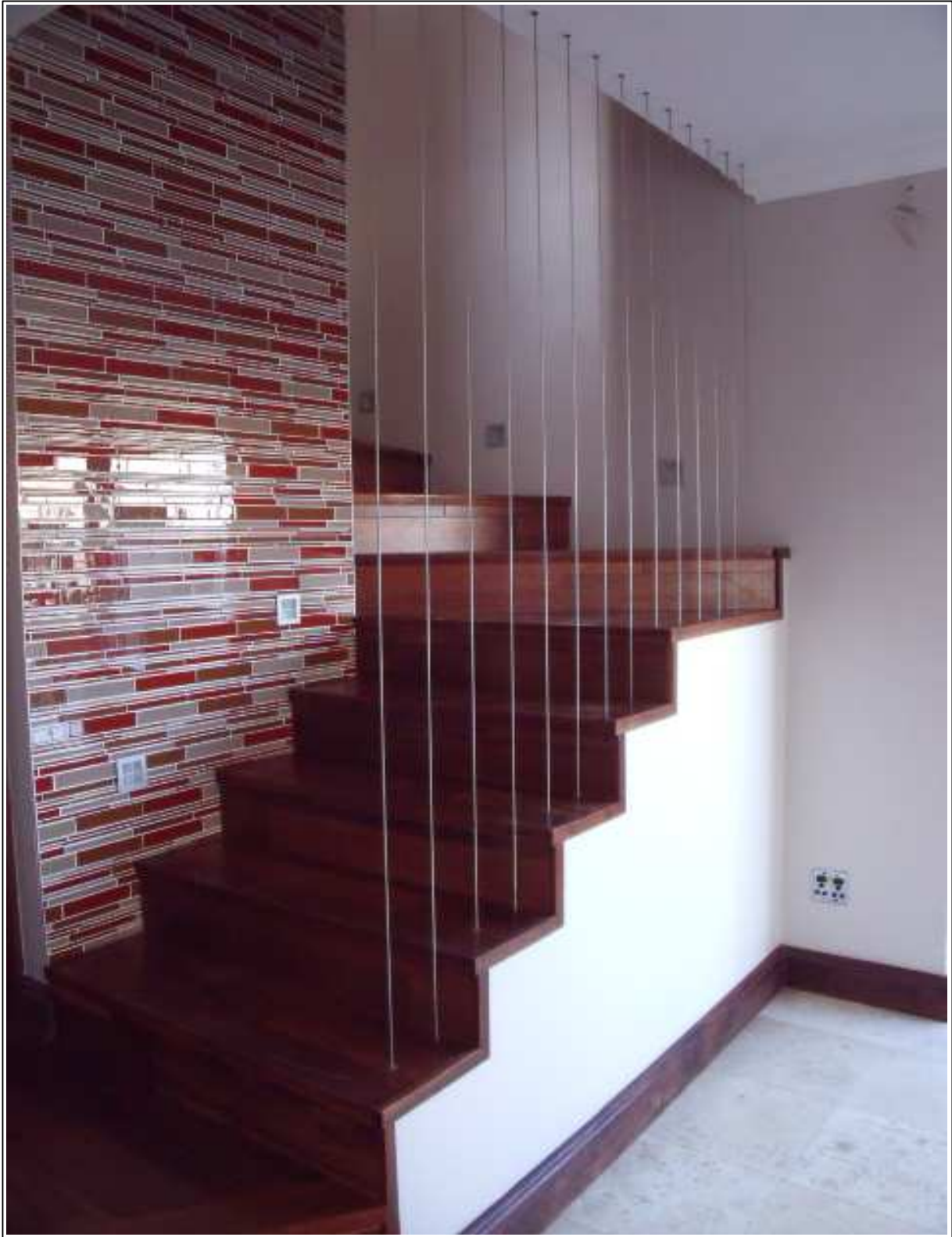
Vertical cables down a stair case
